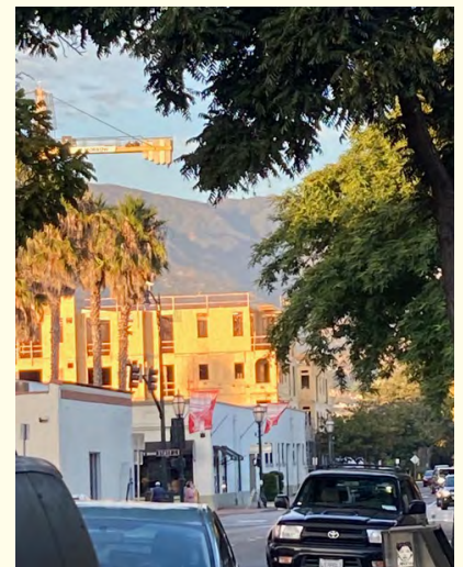
Present-day Santa Barbara: Cranes, construction and congestion. Is this the future we envision?
