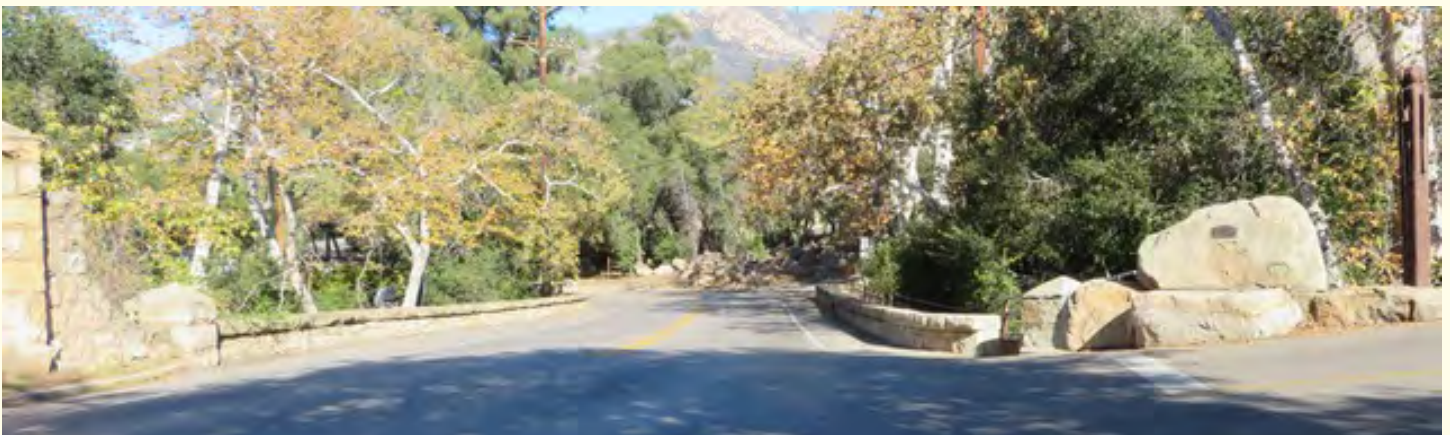
Finished effect that accurately reflects the historic and beautiful entrance into Mission Canyon.
