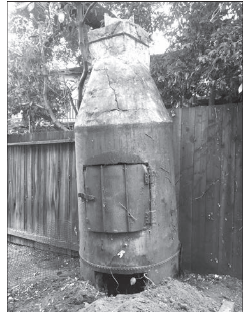
A backyard trash incinerator that was recently demolished (photo courtesy Jennifer Stroh)
